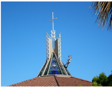
72 panels made up this cone shape piece. 12' tall with a 16' diameter base. Installer had to repel from the top to install the panels.
