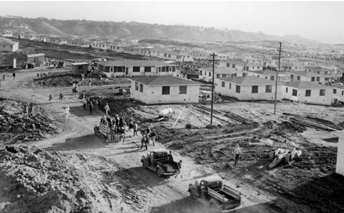
Dirt roads and a sea of newly finished or nearly finished houses were characteristic of Linda Vista during 1941-42.
